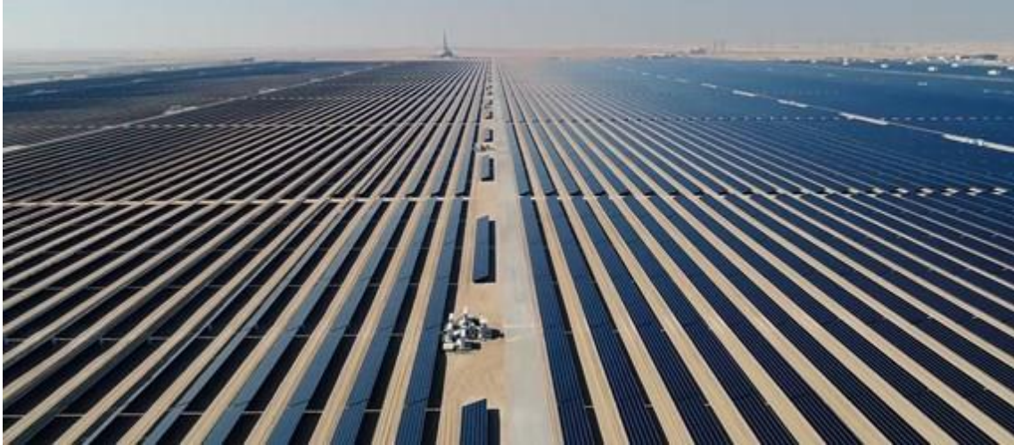
Figure 20. Mohammed bin Rashid Al Maktoum Solar Park, the source of solar electricity for EGA’s CelestiAL solar aluminium [22].
